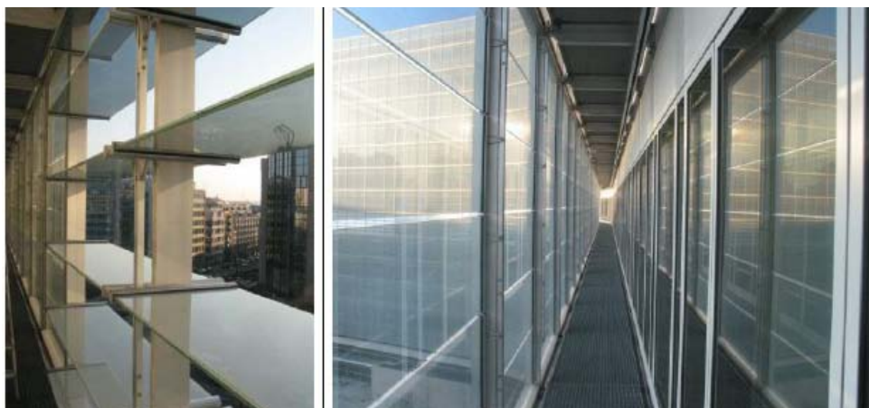
Fig. 29 Ventilated double façade with louvers, a: View of the louvers in horizontal position, b: View of the large cavity and the louvers in vertical position, Berlaymont 'building' Architect : Berlaymont 2000 s.a., P. Lallemand, S. Beckers
