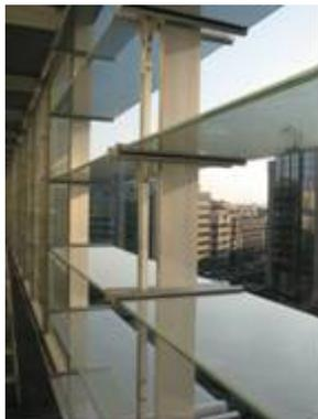
Figure 3.18 View on the louvers in horizontal position.
