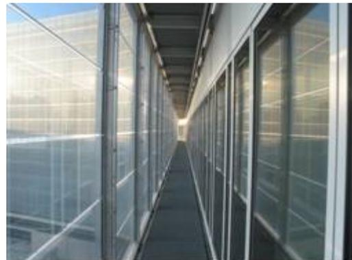
Figure 3.19 View on the cavity with louvers in vertical position.
