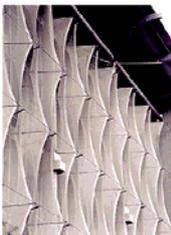
Figure 3.8 Sail-like shading devices on the north elevation of the Phoenix Public Library
