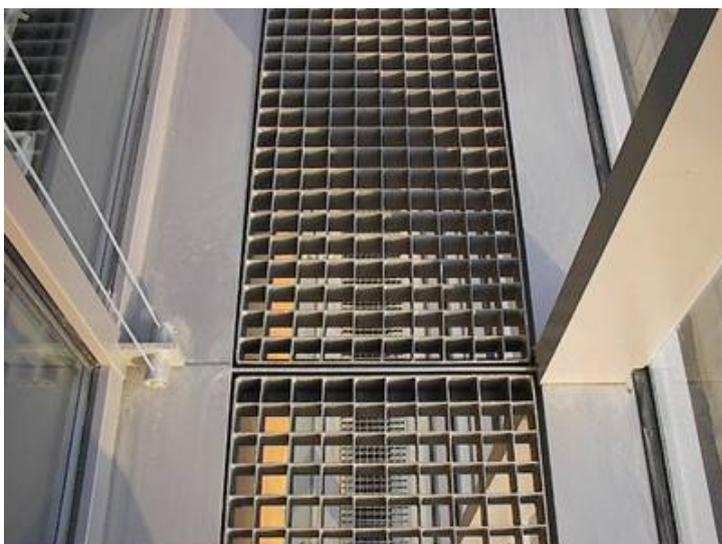
Figure 3.30 View of the walkway through which air is extracted.
