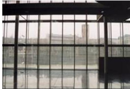
Figure 3.16 Glare through light reflection
