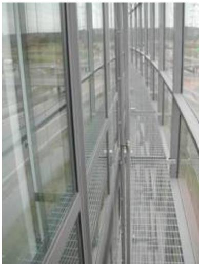
Figure 3.3 Section showing constructive elements of a double skin façade.
